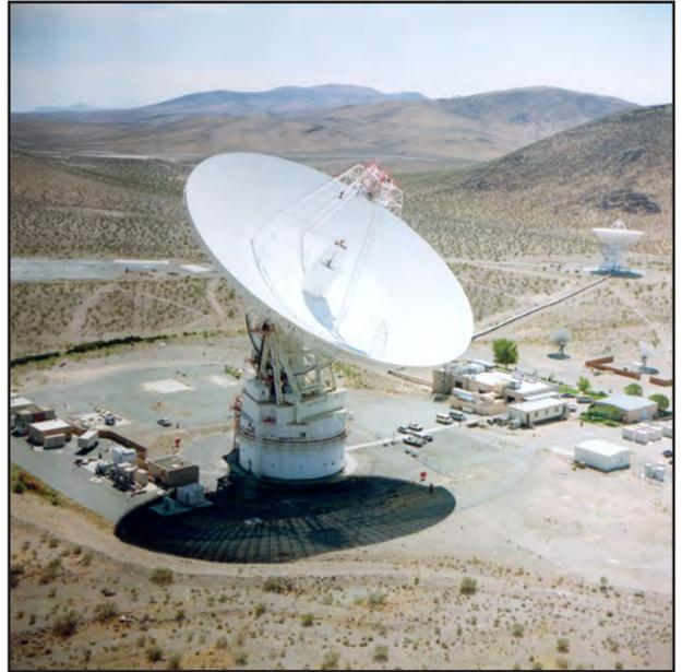
*The seventy-meter antenna located at the Goldstone Complex near Barstow, CA. This is one of the three highest sensitivity antennas for spacecraft tracking located around the world.*
